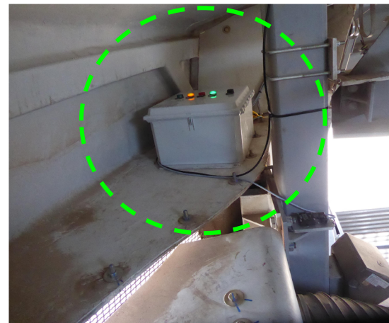
Swarm Edge installed in each of 10 turbines, both GE and Clipper models.
